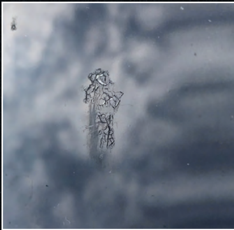
Bat Droppings Stains
