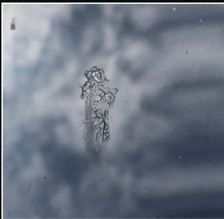
Bat Droppings Stains
